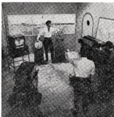
Before automation • Two cameramen and a floor director are required on the scene to put the show on the air. Headsets put them in contact with the director.
