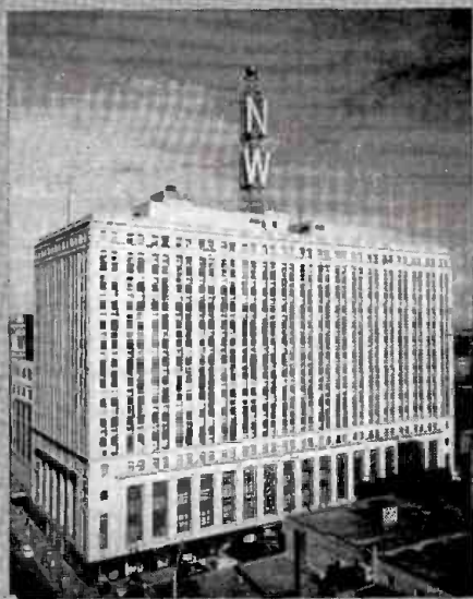
Northwestern Bank Building
